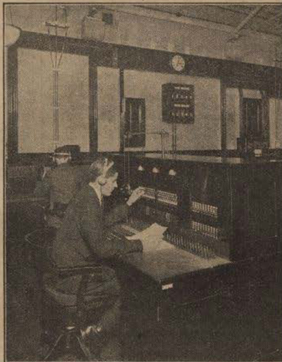
"SIMULTANEOUS BOARD" IN THE CONTROL ROOM OF THE LONDON HEADQUARTERS OF THE B.B.C.
